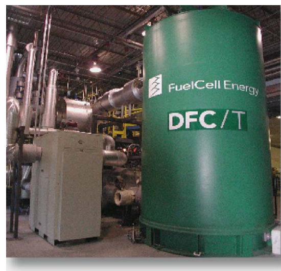
Fig. 2. FuelCell Energy DFC/T hybrid.
